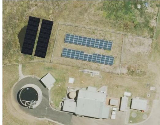
FIGURE 67: BARRABA WTP – 40 kW SOLAR ON WEST-SIDE ADJACENT LAND W/ 100 kWh BESS
