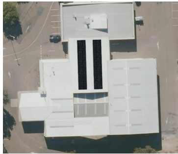
FIGURE 81: FLYNN STREET DEPOT – 42 kW FLUSH-MOUNTED ROOF SOLAR PV SYSTEM
