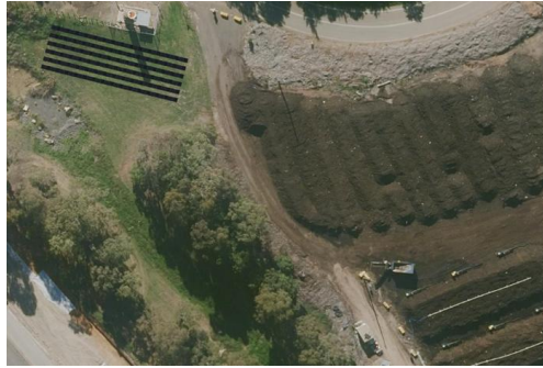
FIGURE 105: FOREST RD LANDFILL – LANDFILL – 45 kW GROUND-MOUNTED ROOF SOLAR PV SYSTEM
