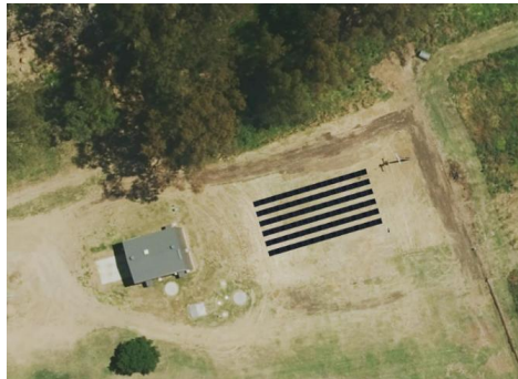
FIGURE 71: NAMOI PUMPING STATIONS – 30 kW GROUND-MOUNTED SOLAR PV SYSTEM W/ 45 kWh BESS
