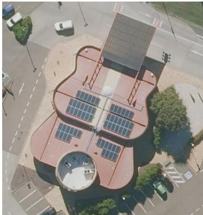
FIGURE 34: AUSTRALIAN COUNTRY MUSIC HALL OF FAME ONSITE SOLAR
