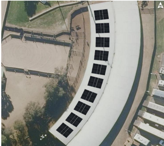
FIGURE 8: AELEC – 50 kW SOLAR ON CATTLE HOLDING AREA
