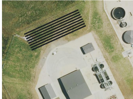
FIGURE 62: MANILLA WTP- 84 kW SOLAR ON NORTH LAWN W/ 120 kWh BESS
