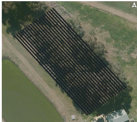
FIGURE 46: CALALA WTP – 400 kW GROUND-MOUNTED SOLAR PV SYSTEM B/W THE PLANT AND CALALA STORAGE DAM
