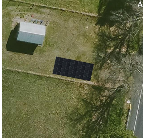
FIGURE 76: NEMINGHA PUMPING STATION – 12.5 kW POLE-MOUNTED SOLAR PV SYSTEM W/ 30 kWh BESS
