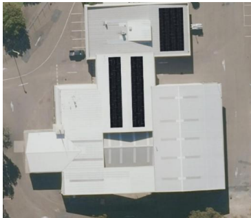
FIGURE 83: FLYNN STREET DEPOT – 68 kW FLUSH-MOUNTED ROOF SOLAR PV SYSTEM W/ 146 kWh BESS
