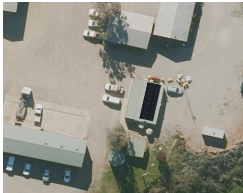
FIGURE 106: FOREST RD LANDFILL – NORTH RESERVOIR – 10 kW FLUSH-MOUNTED ROOF SOLAR PV SYSTEM
