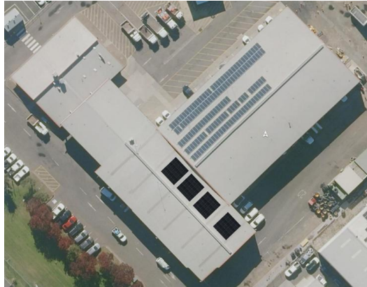
FIGURE 88: LOCKHEED STREET DEPOT – 30 kW ADDITIONAL FLUSH-MOUNTED ROOF SOLAR PV SYSTEM / 50 kWh BESS
