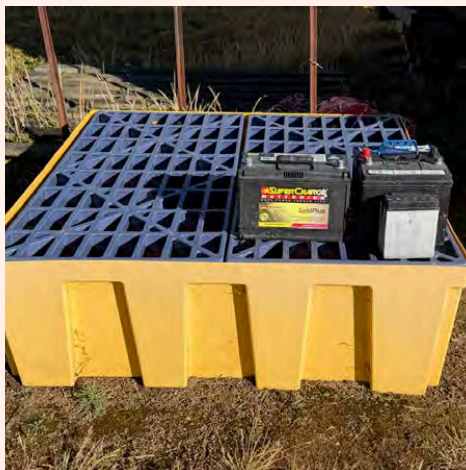
Barraba - spill pallet for batteries
