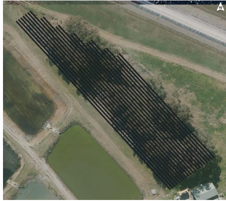
FIGURE 48: CALALA WTP – 622.5 kW GROUND-MOUNTED SOLAR PV SYSTEM B/W THE PLANT AND CALALA STORAGE DAM W/ 700 kWh BESS
